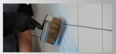
CN 94 is solvent free and contains a **blue pigment to control the application more easily.** For absorbent surfaces only the amount needed to cover the whole surface should be used, and for non-absorbent surfaces as much as will work.
