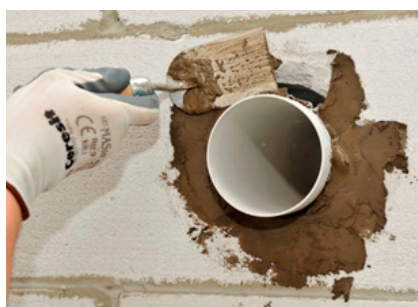
Assembly with Ceresit CX 5 EXPRESS mortar (substrate prewetted)
